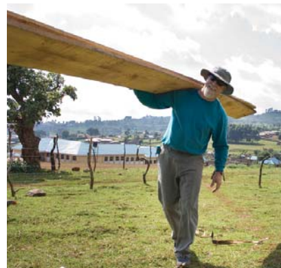
Kent Boles of Sisters assists with school construction.
