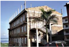
Dining Hall and Library on Gaba Campus
